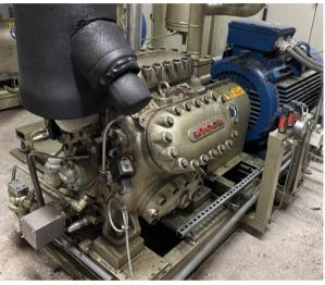
Very nice complete NH3 /Co 2 plant . In the Nh3 side are 2 very well maintained Mycom 200 VLD Vi 3.6 driven by 315 kW E-motors. On the Co 2 side are 3 Mycom C6HK piston compressor installed. This plant was started in 2013. And will be dismantled in approx. September 2025.
