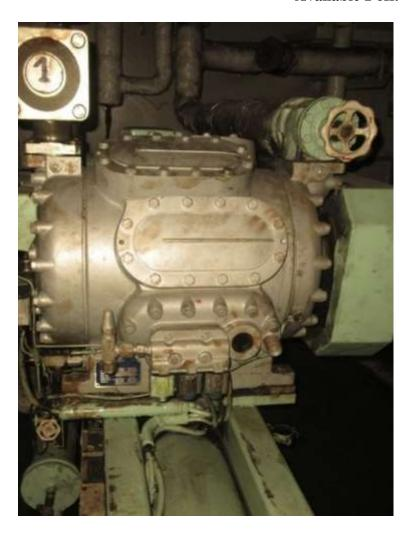
1 pc Sabroe CMO 28 compressor block suitable for Freon. available Year of build 2019.
