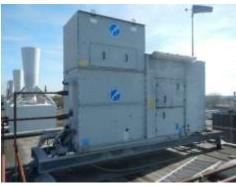
**Available:** Grasso Glycol chiller till -45 °C, Based on a Frequency driven Grasso RC7212E incl Frequency convertor and Baltimore condenser. The E-motor is 75 kW. Refrigeration : 109 kW Complete control cabinet . Dimensions: 5000 x 2600 x 3000 mm Weight: 6000 kg
