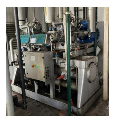
Sabroe Twin unit based on Sab 128 HF compressor, controlled by 2 Unisab PRO II controllers. The E-motors are 110 KW Schorch. The unit was running on NH3. Freon is also possible.
