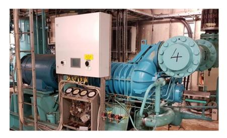
Stall SVB75 models are heavy duty - Strong due the radial youral bearings and thurst bearing construction for the Axial play. Oil pump is mouted direct on the compressor . Still all spareparts are available.
