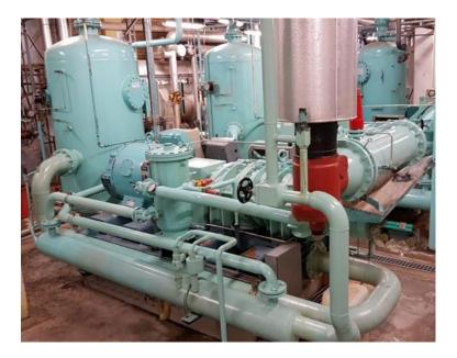
Stall SVB67 compressor block are suited with journal and thrust ball bearing for long life operation. All spare- parts asre still availble – the oil pump is direct mounted on the compressor .
