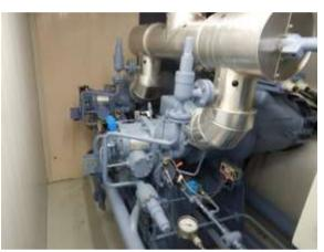
Very nice maintained machine room NH3 pump system. Complete build in a 40 ft container. Air condenser Thermofin type: TACH 080-1-26-AL – oil cooler air cooled: Thermofin TDH 050.1-22.AN (D5) H4-12P. Witt liquid separator with Witt NH3 pumps. Complete control panel Siemens S7 PLC.
