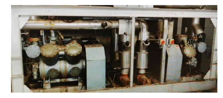
On skid contains 2 pc V- Belt driven Grasso RC12 compressor units. The RC412 is suited with a 90 kW E-motor, the RC312 is suited with a 75 kW E-motor. The compressors are constructed in 1996. In the skid are 2 NH3 pumps present
