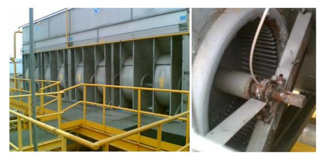
Example: Installation in hot sandy country on the fan bearings of a refrigeration condenser.
