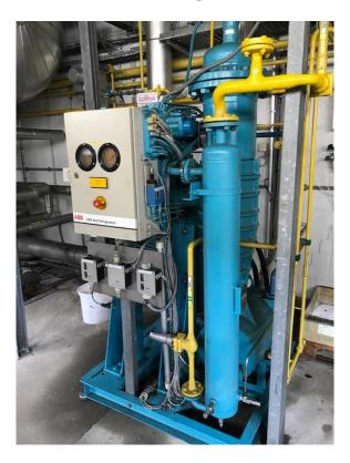
Very well maintained Stall Compact  $R59-small\ Foot\ print$  - Stall was one of the first developers of the compact screw compressor unit – The unique design was the oil separator , which was based on centrifugal forces.
