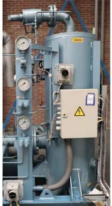
The oil separator is GEA version with oil separator elements in last stage.
