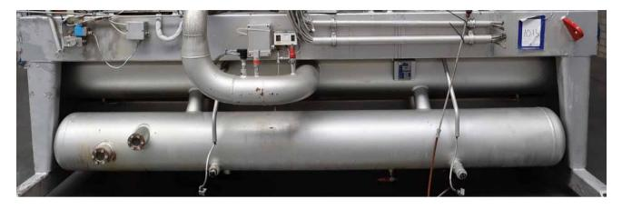
The unique construction of the Sabroe oil separator is the oil buffer tank, which is below the original oil separator. The oil will be collected in the lowest tank.
