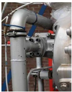
On the Compressor block is a direct drive full flow oil pump mounted . As soon as the compressor is running the pre-lube pump stops and the Full flow oil pump takes over the duty of pressurizing the lubrication oil.
